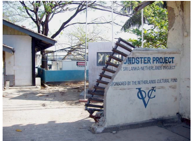
The entrance of the MAU after the Tsunami
